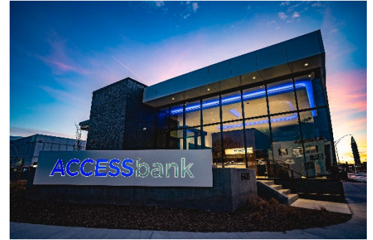
The new ACCESSbank location in Omaha.
